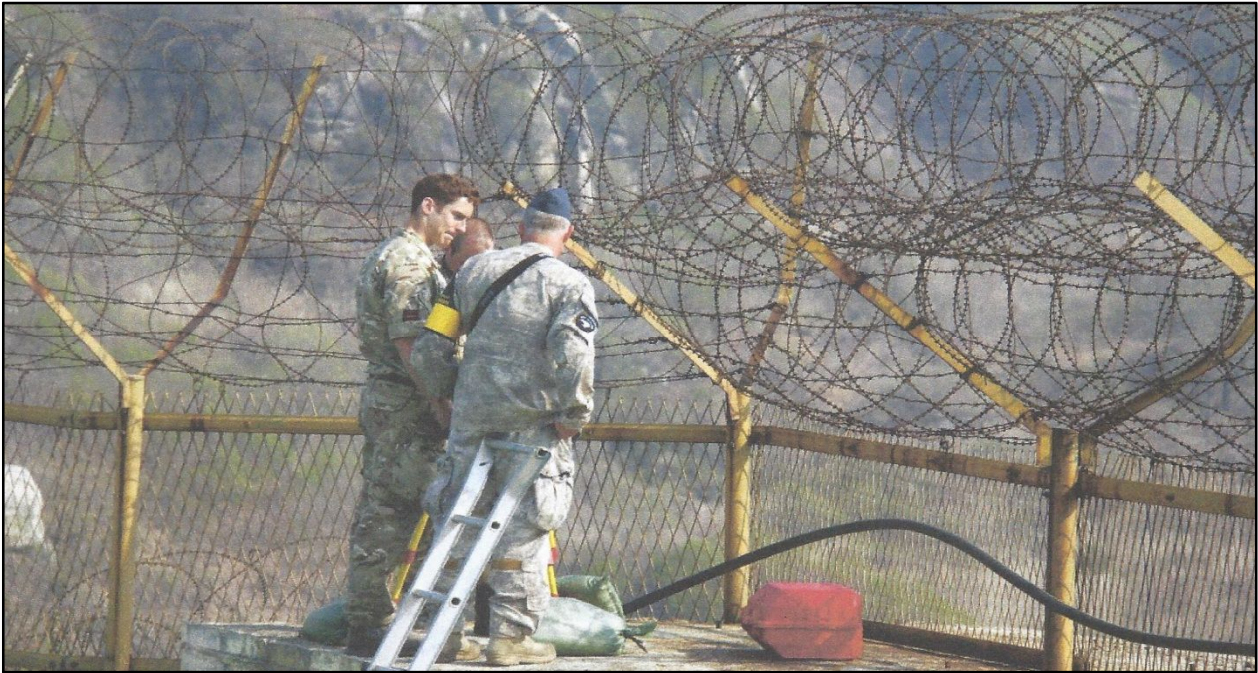
A less than ideal set up in close proximity to a chain fence and coils of razor wire
